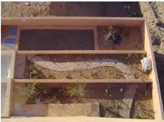
Grey-water tank and planned water treatment (plants still to be introduced in the gravel bed)
